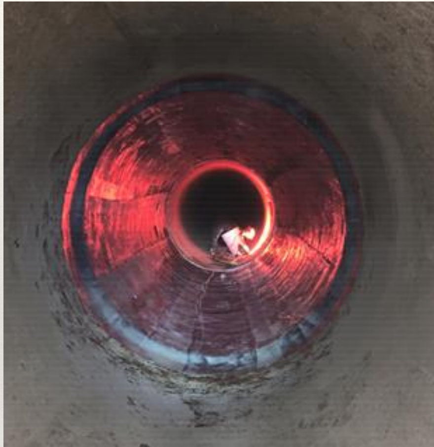
Proactive Internal Carbon-Fiber Repair of 54" PCCP
