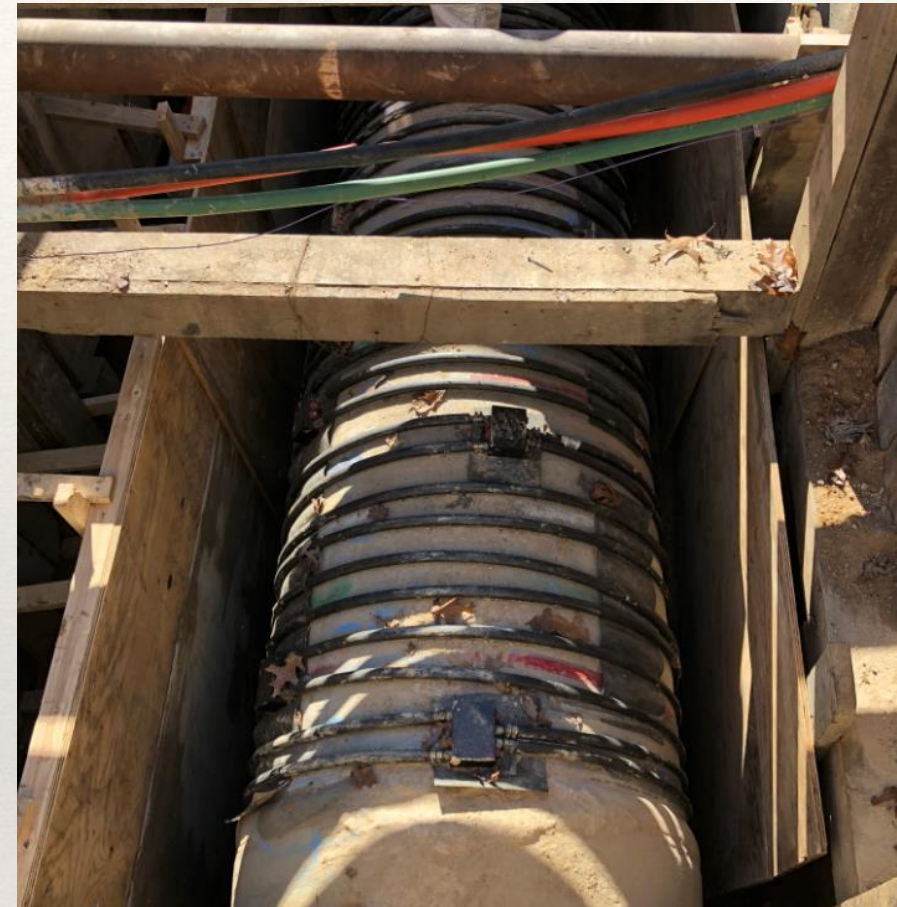
Proactive External Post Tension Tendon Repair of 48" PCCP
