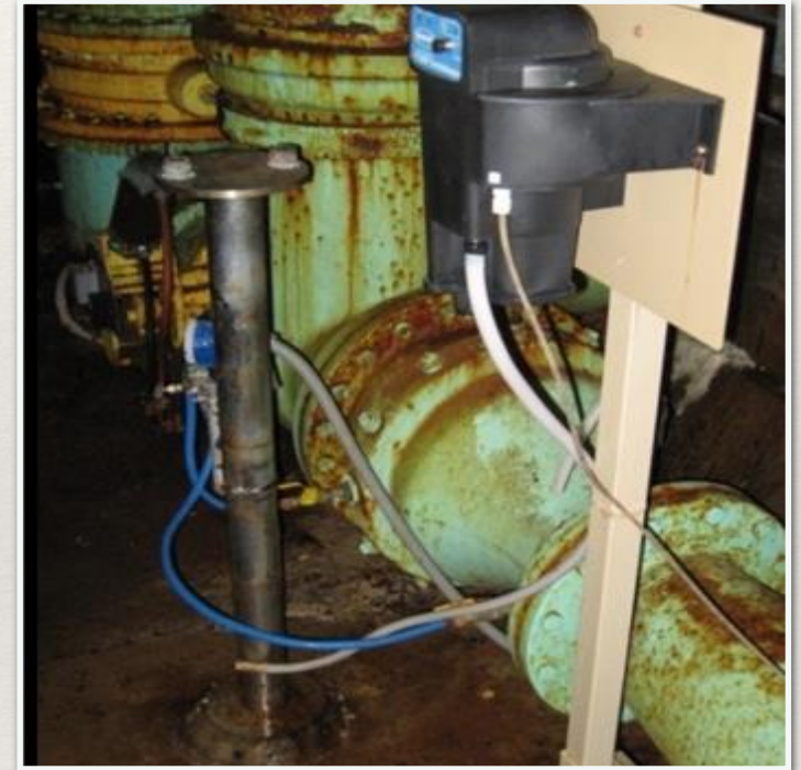
Existing Filter Piping Conditions
