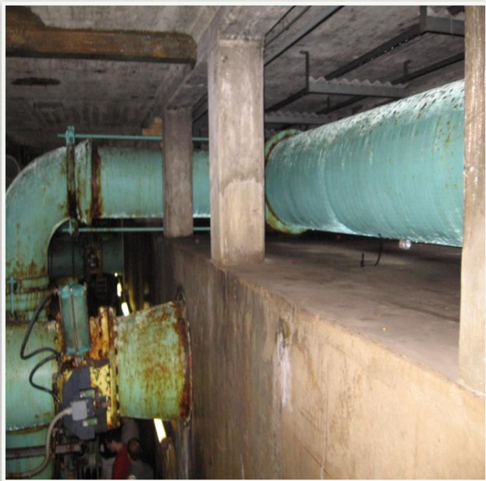
Hydraulic Valve Actuator Corroded Leakage
