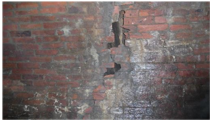
Current Condition Missing Mortar and Bricks
